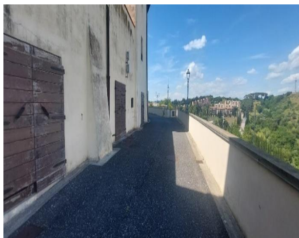
27 Flat and asphalt path to reach the terrace
