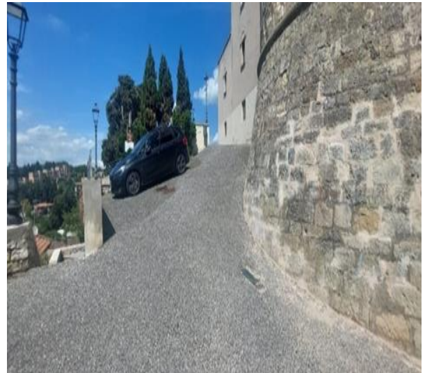
35 descent ramp to the entrance to the castle
